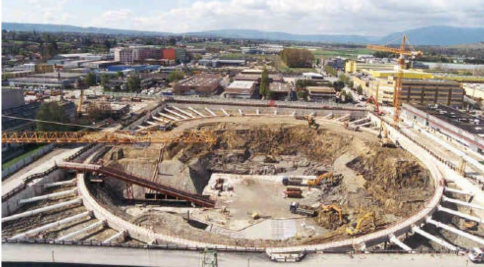
Figure 1: Excavation during the earthworks.
